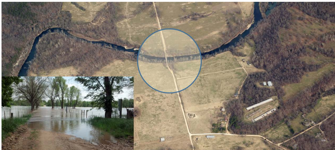
Fisher Ford Bridge STP-A project
