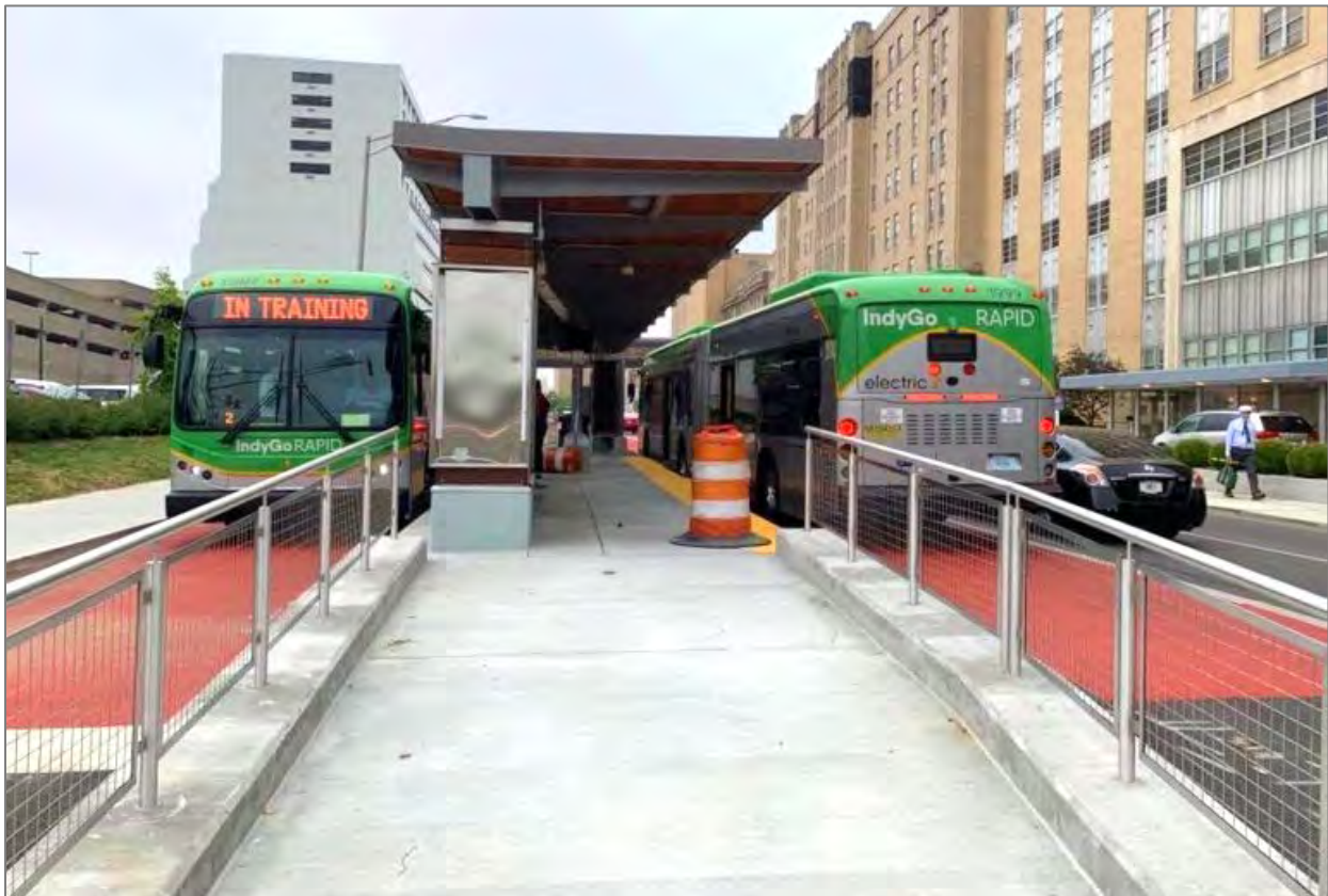
Figure 94 IndyGo Red Line BRT Station and Bus-Only Guideway, Indygo.net
