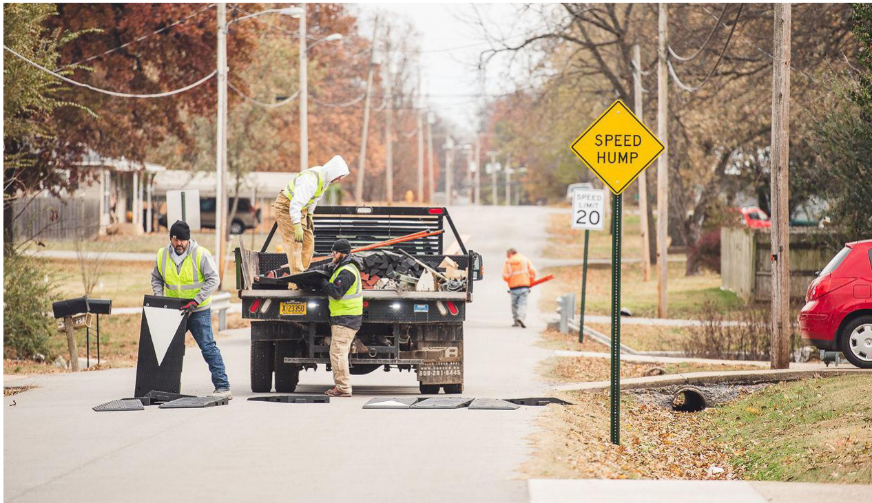
Siloam Springs Neighborhood Greenway Installation (credit: Trailblazers)
