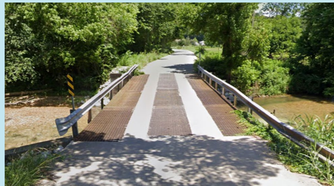
Wagon Wheel Road Bridge Replacement
