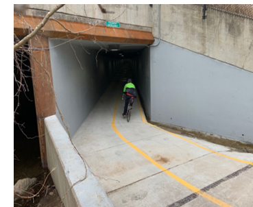
Improved tunnel under the Fulbright Expressway on Razorback Greenway in Fayetteville.
