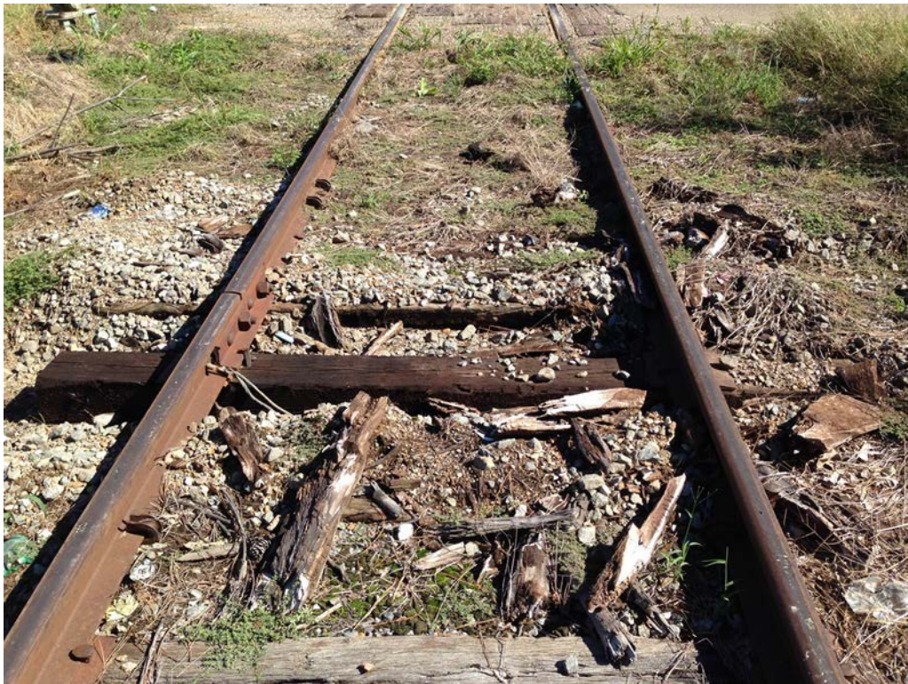
Figure 9-1. Segment of Excepted Track in Arkansas
