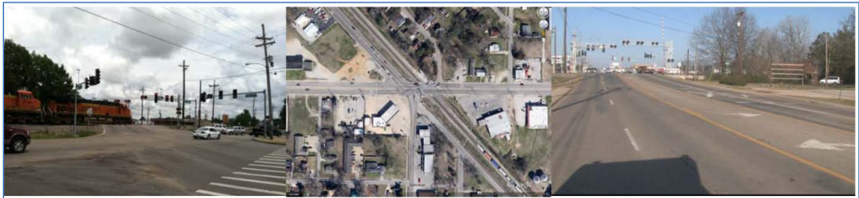
Figure 11-1. Highway 18/BNSF Crossing in Jonesboro
