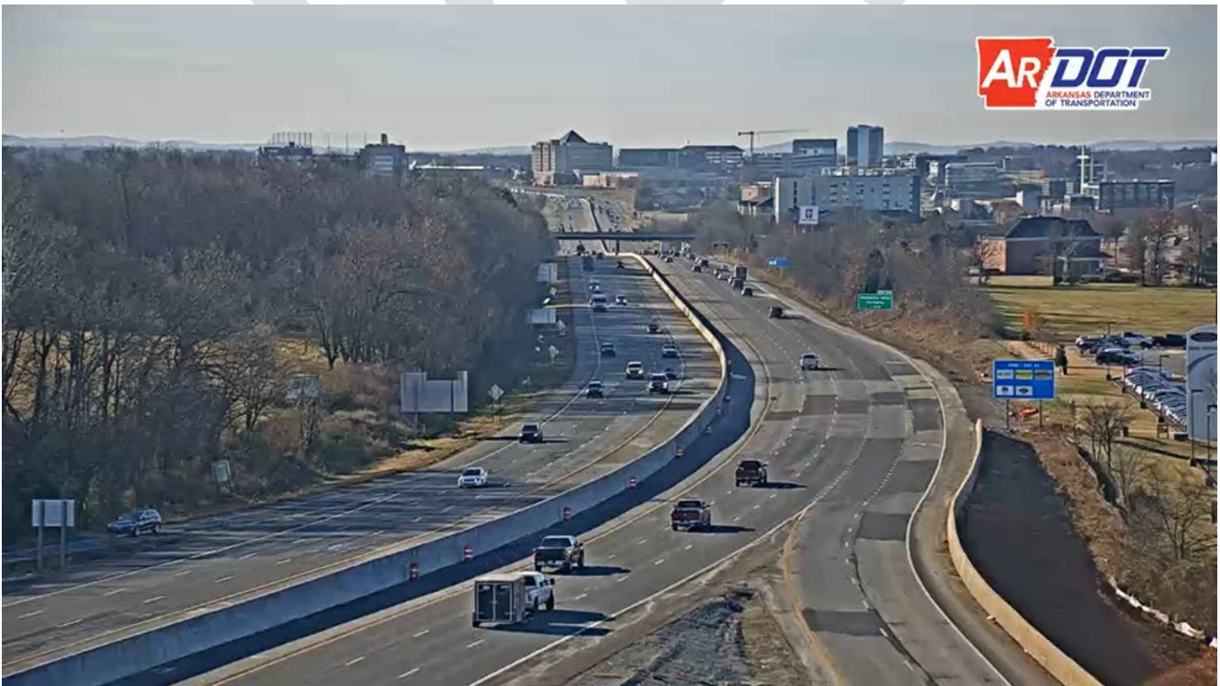
I-49 View from Walton Blvd/Walnut Street Bridge in Bentonville/Rogers
