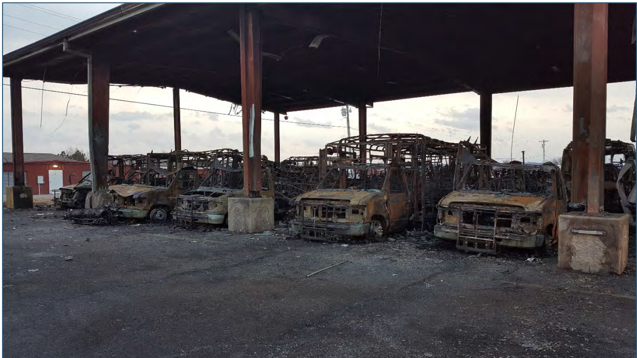
Figure 1.2 Buses Destroyed by January 10, 2017 Fire
