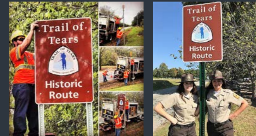
ArDOT sign installation crew
